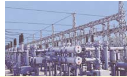
36 ~ 72.5kV GIS (Gas Insulated Switchgears)
