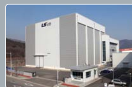
HVDC Plant, Busan
