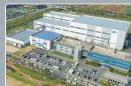
Power TR Plant, Busan
