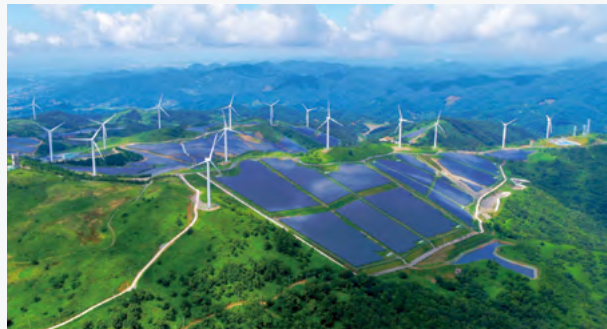
Photovoltaic Power Business in Yeongam
