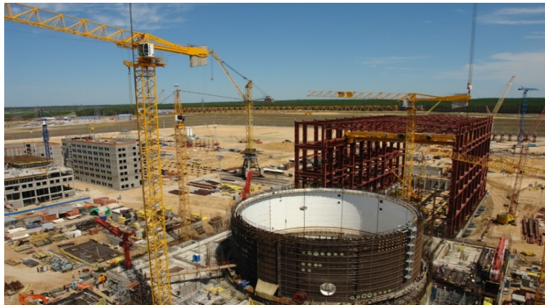
Concrete building electric room (Stick Built type)
